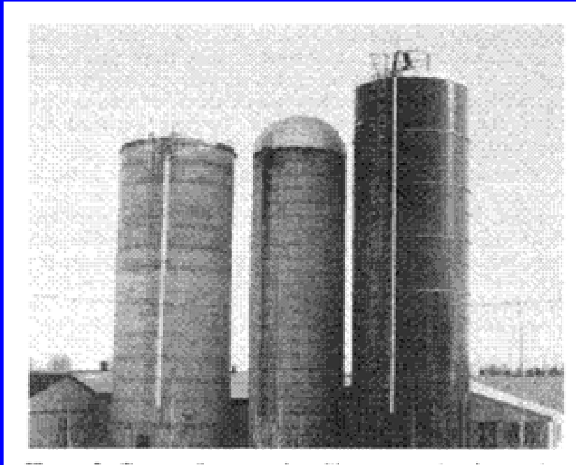
Figure 2. Tower silos may be either conventional open-top (usually concrete, cast-in-place or pre-cast stave), or oxygen limiting (usually concrete or glass-lined steel).
